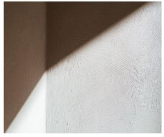
CANVAS FINISH The Canvas finish is made by using a wide paint roller to apply the Marble Paint in long strokes across the surface. This technique imparts a naturally dappled effect that gives textural depth when viewed up close, while the entire surface appears more uniformly structured from afar.
