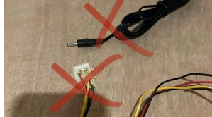
Figure A-7: No connection of wires
