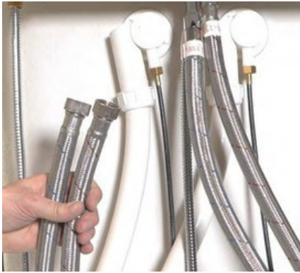
Connect to Shut Off Valves (not included)
