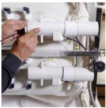
T-Type four (4) 2" drain ports allow for the drain pipe to installed either be in direction.
