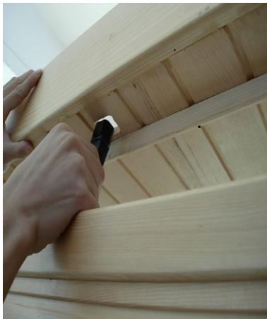
FIG-12 Slip cords/wires through corresponding holes
