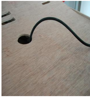
FIG-18 Pull Power Cord through Roof Cover
