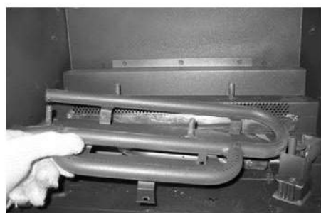
Burner Removed
