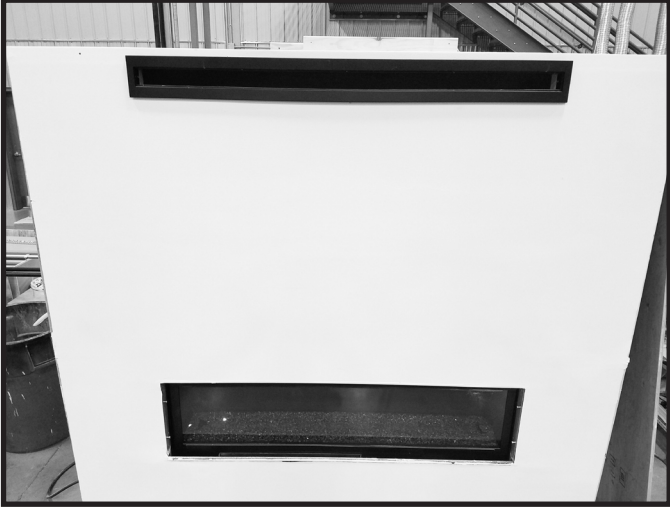
Figure 6 Vent Cover Installed
