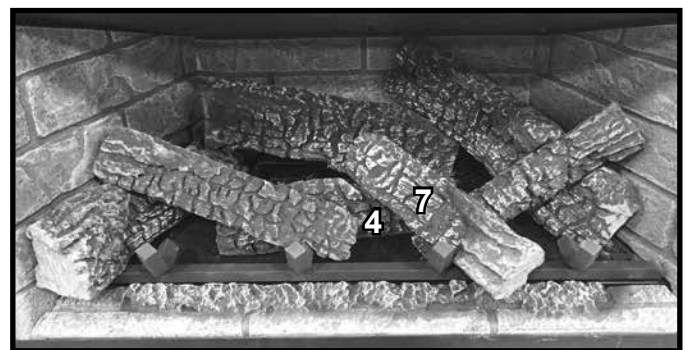
Figure 10. Log #7 Installed
