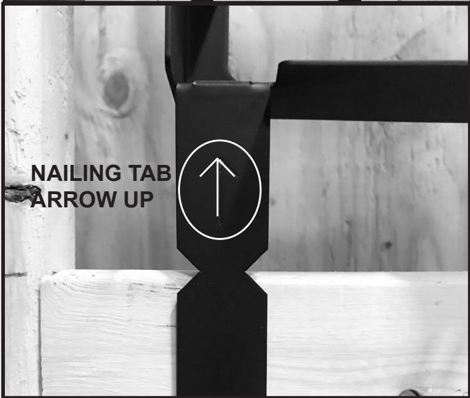
Figure 5.13 Side Discharge Assembly Nailing Tab Orientation
