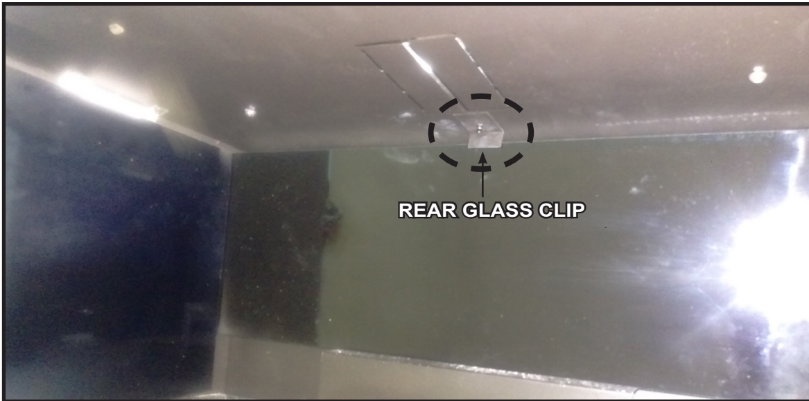
Figure 6. Install Rear Glass Panel
