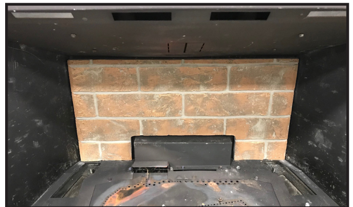
Figure 5. Back Refractory Installed
