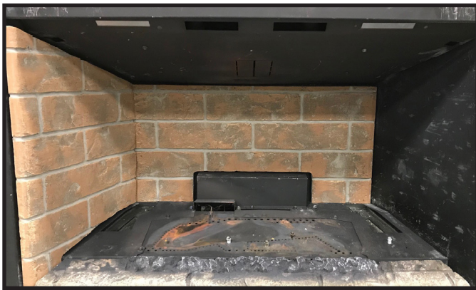
Figure 7. Left Refractory Installed
