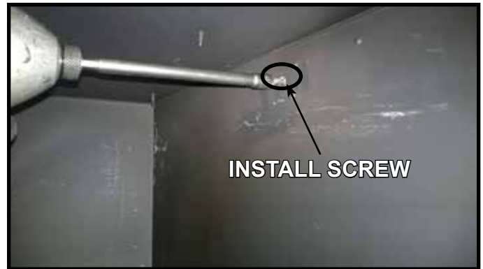
Figure 1. Remove Fiber Refractory Brackets. Install Screw.
