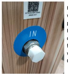
Hang on to the Caps and Plugs that come with your Cold Plunge! The Caps are great for protecting the threads on the Inlet and Outlet Fittings when the Cold Plunge is not connected to a Chiller. The Plugs are helpful for isolating the Cold Plunge from the Chiller when replacing the Filter or cleaning the Chiller Strainer.
