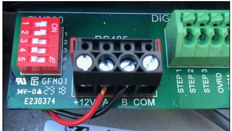
Figure 10 - New Wires from Circulation Pump to Heat Pump and DIP switches
