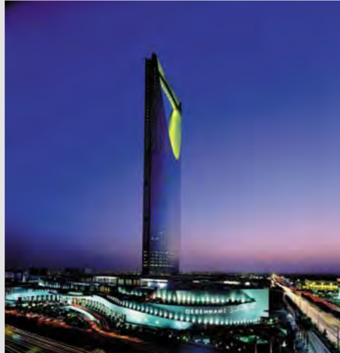
Kingdom Tower, Riyad, Saudia Arabia
