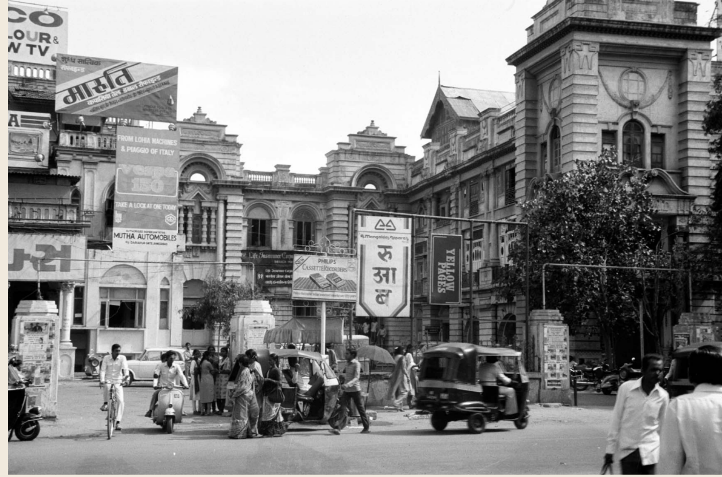
The building was tenanted to many entities including Government offices, private offices, clinics and a restaurant. The family members account offices and some entrepreneurial ventures started by individual members also operated from here.
