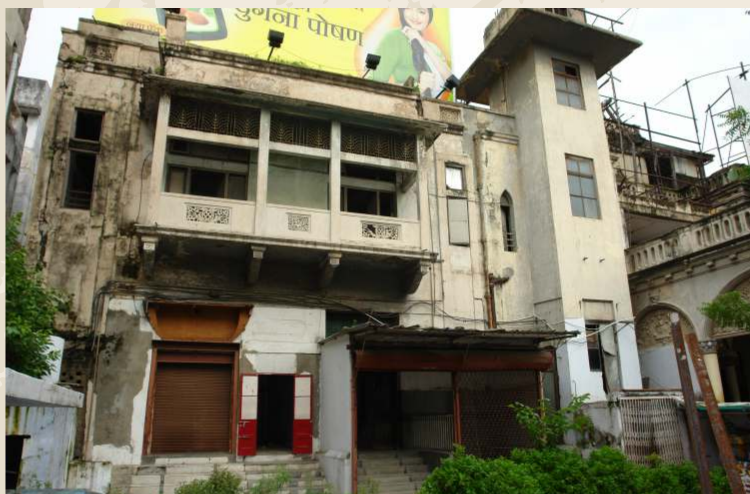
CG wing facade in 1995. An empty shell where once there was a home.
