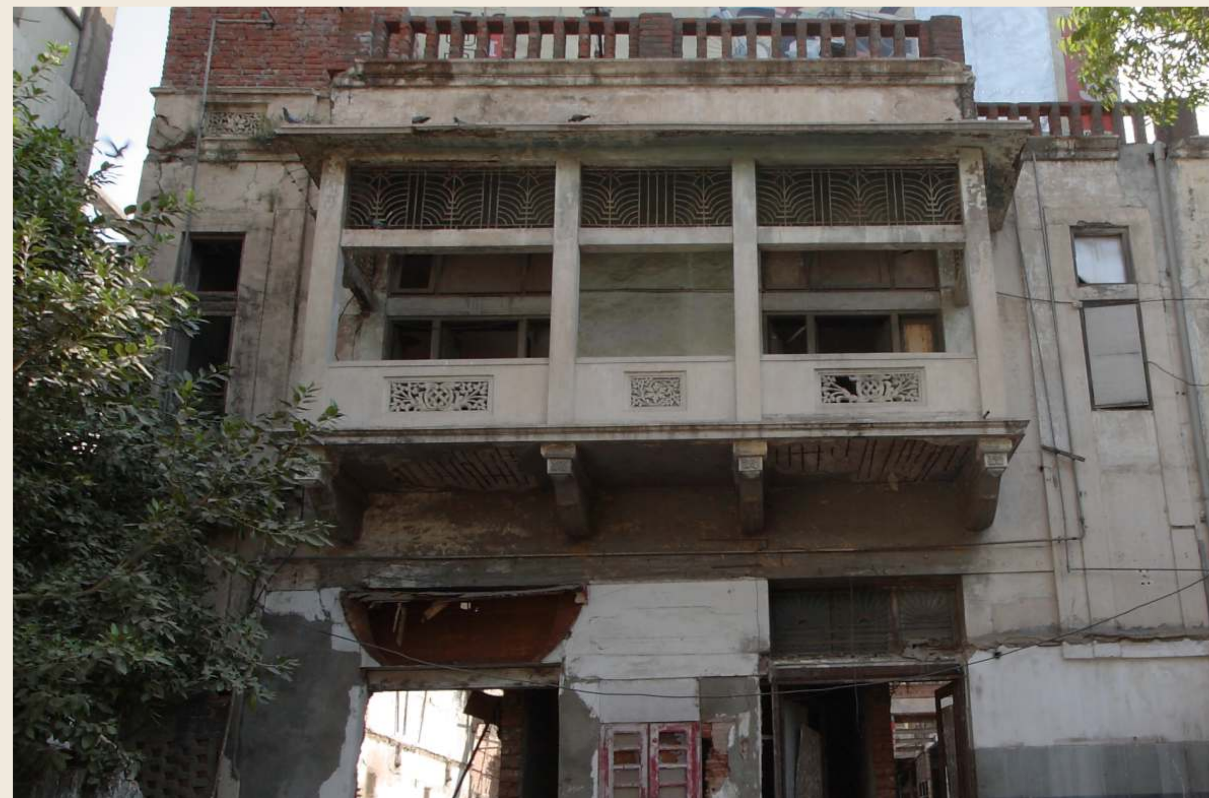
State of CG Wing before renovation.
