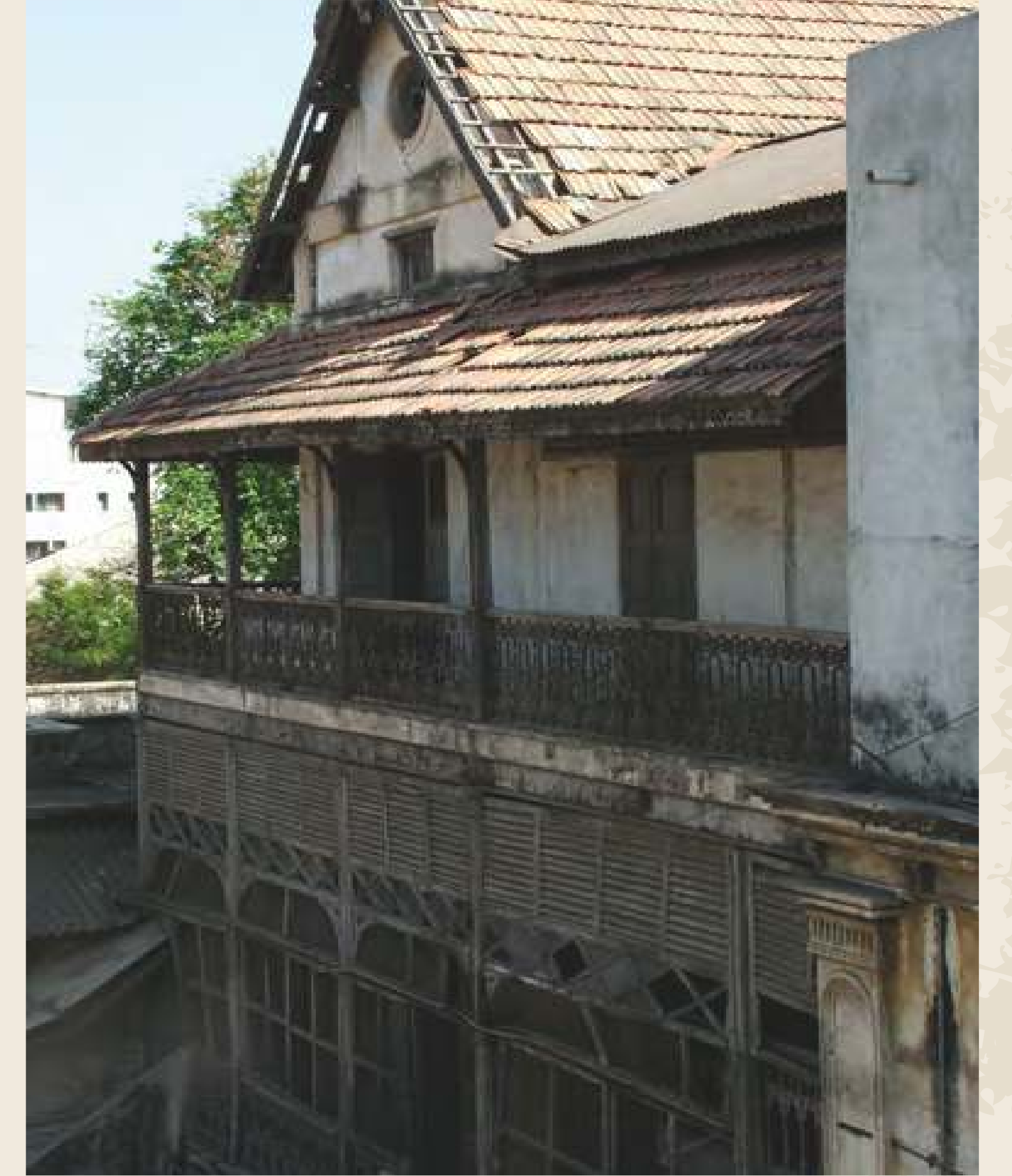
State of the woodwork before renovation.
