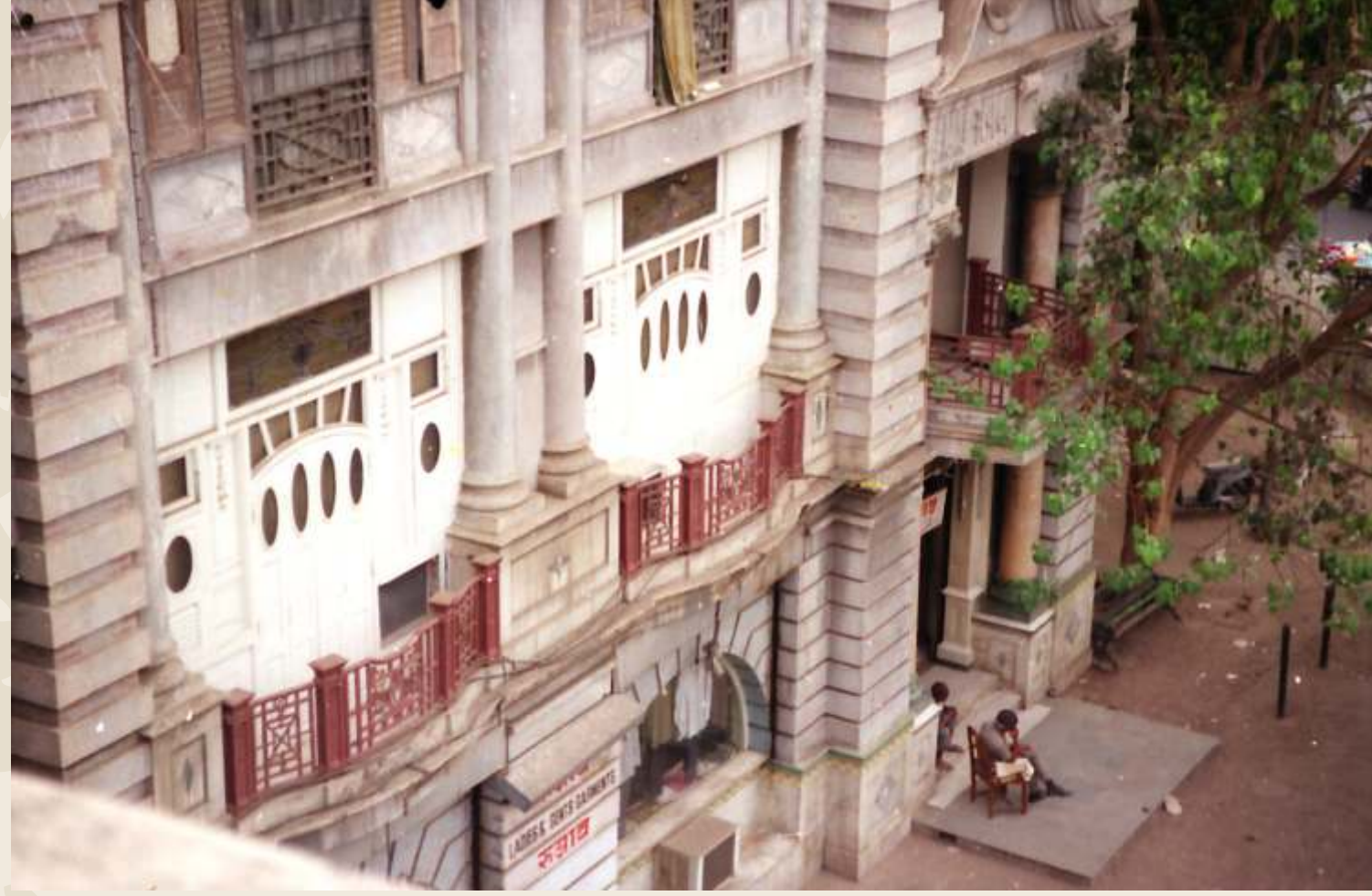
AM Garment Shop on first floor and Ruab Denim Store on the Ground floor of the house. Aryodaya Mills was amongst the first mills to make denim in India.
