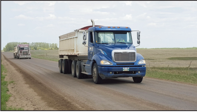
Figure 2. Curries Landing haul road near Brandon, Manitoba after stabilization using clay-rich soil and organic catalysts. Photo: Cypher Environmental.
