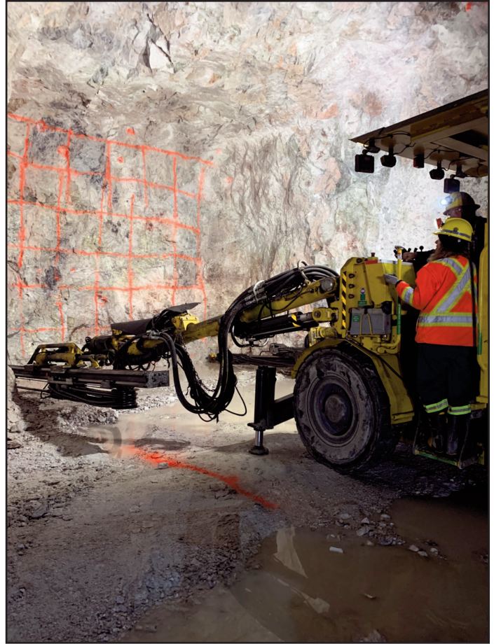
Figure 3. Underground mining operations at the Tanco Li-Cs-Ta mine, southeastern Manitoba. Photo: T. Martins.
