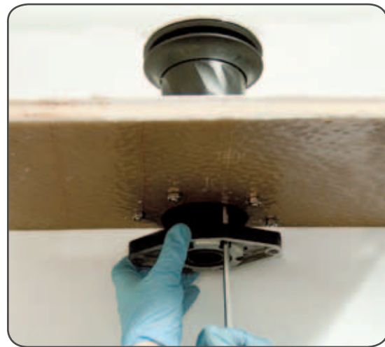
2. Tighten the six screws (8 Nm/ 71 in-lb)
