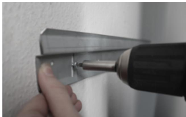
**3)** Make sure that the carrier is level, by using the spirit level and adjusting the carrier.
