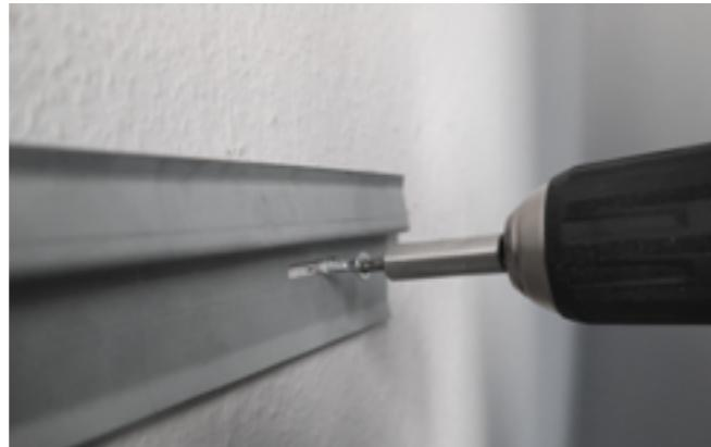
**2)** Screw the second screw in the horizontal hole of the carrier.
