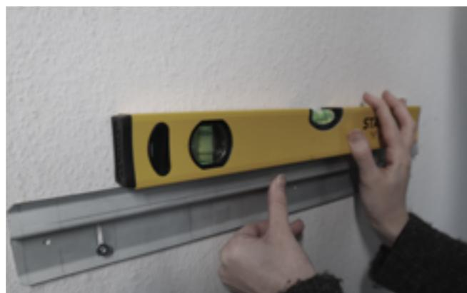
**4)** Measure from the top edge of the carrier and down to the top edge of the second carrier.
