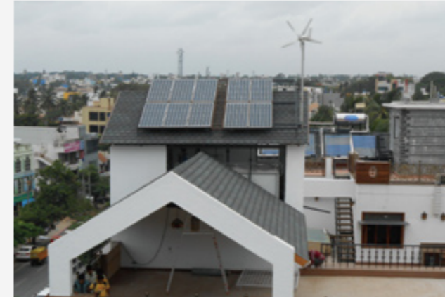
1.5KW wind solar hybrid off-grid power system for residential - Bangalore India - 2011
