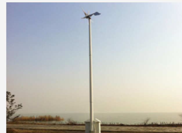
HY-1500 grid-tie system with 10.4m hydraulic tower installation - Sweden 2012
