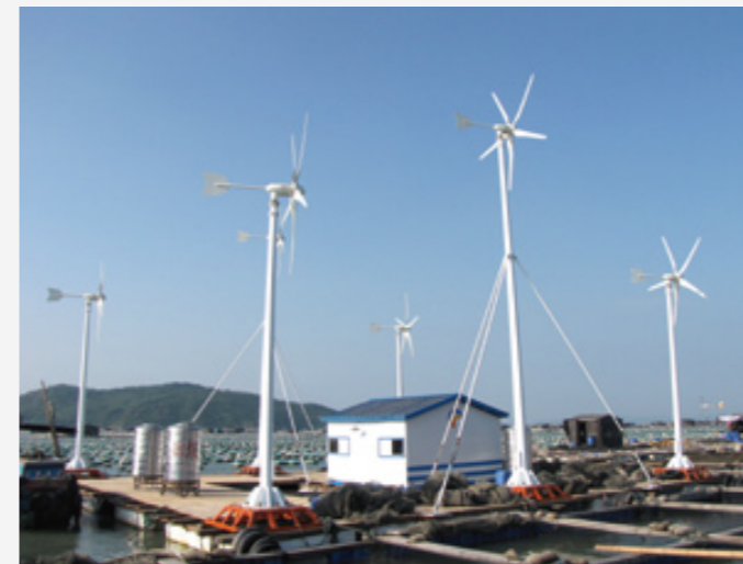
18KW wind powered stand-alone sea water desalination system - Bureau of Fishery, Fujian 2008
