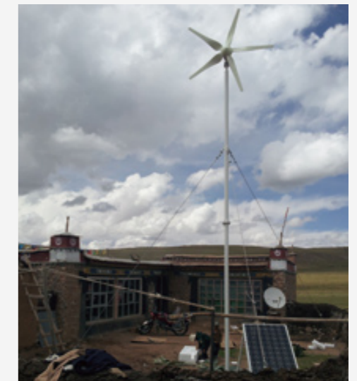
800W wind solar hybrid off-grid power system for remote village – Tibet 2006
