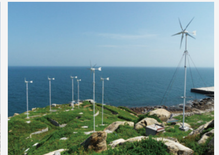
21KW wind powered stand-alone sea water desalination system – Nanpeng island, Shantou 2010
