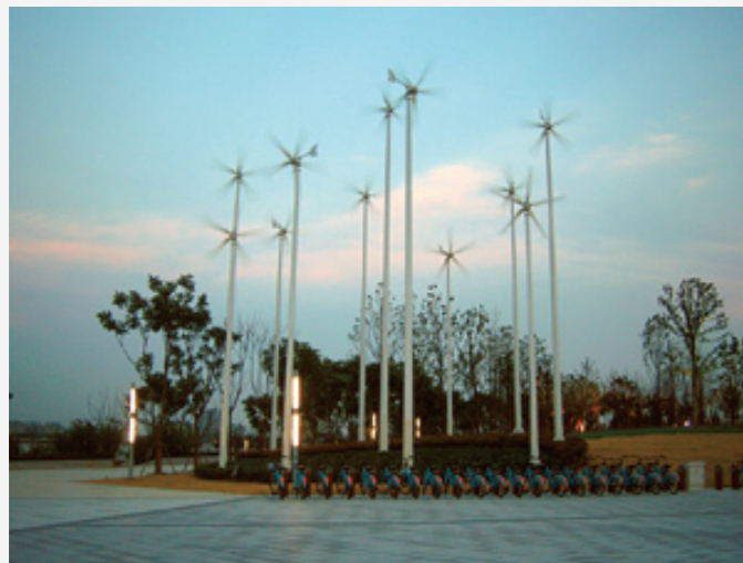
Total 33KW wind power array off-grid power system for eco-park lighting – 11pcs of HY-3000 wind turbine created off-grid system to power all lights of Binjiang Eco-green park, system is designed and constructed by HYE– Shanghai 2010
