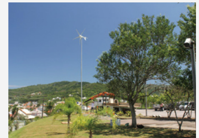
HY-3000 grid-tie system with 13.4m hydraulic tower installation - Florianopolis Brazil 2010
