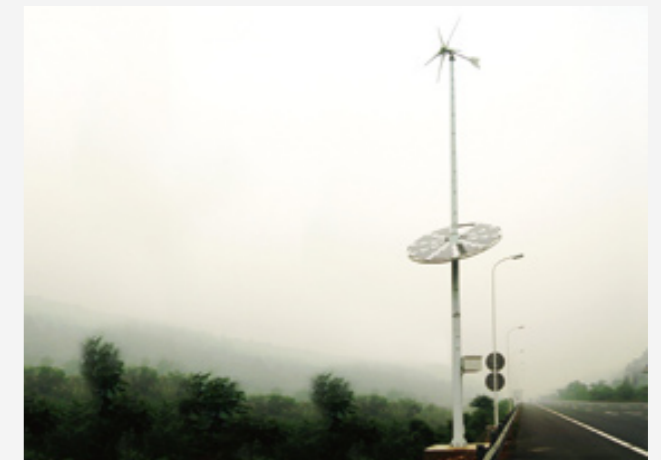
Sky Driven system power 7pc 85W LED street light – suburb Guangzhou 2011
