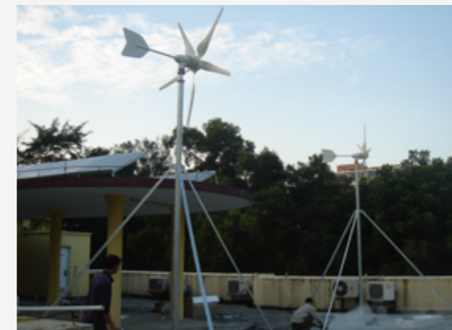
4KW wind solar hybrid off-grid power system for small business enterprise rooftop – South Korea 2010
