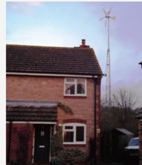
HY-1000 grid-tie system with lattice tower - Liverpool UK- 2009
