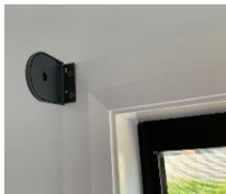
Fit idle end bracket
