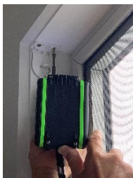
Fit Clutch bracket
