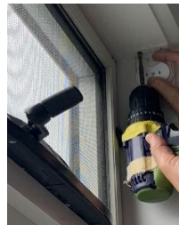
Measure the blinds width, fit Idle end bracket on the other side.
