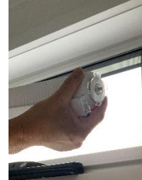
Insert idle end plug into idle end bracket
