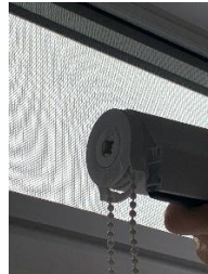
Insert clutch side into clutch bracket
