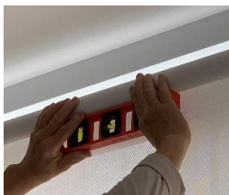
Using spirit level to check if the blinds fitted on the same level
