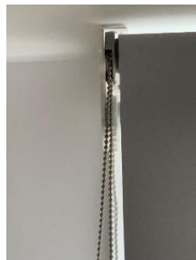
Insert idle end plug into upper idle end bracket ( blackout blinds )
