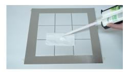
4. Press the trigger to squeeze the grout out to get rid of the initial 1 foot material, which is not mixed evenly and not advised to grout the joint.
