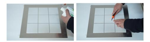
1. Take off the cap and cut cartridge seal. Cut the nozzle outlet to meet the joint width. A vertical cut is advised.
