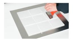
4. Leave the site as it is after the grout lines are pressed and shaped, until the material cures. Do not use water to scrub the excess which is not water cleanable. It normally takes around 4 hours in hot and dry weather for the material to set. You can finger touch and feel its hardening. After it sets, scrape the grout residue, clean the floor and the work is completed.
