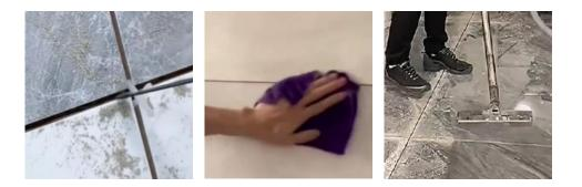
1.A good preparation makes a half success. It's very important to clean the tile joints thoroughly before the grout work. Use the hook, knife or scraper to clean up the mud, sand and spacers in the gaps. Wet wipe and vacuum the tile surface.
