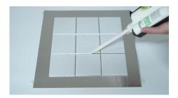
1. Match the nozzle to the tile joint. Press the trigger. Move the gun slowly and steadily to squeeze the grout into the joints.
