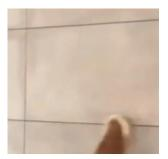
2.Spread the cleaning paste (working as grout release agent) smoothly and lightly over the tile joint horizontal surface (Note: Do NOT spread the paste into the joints, otherwise it may affect the bonding of the grout). It facilitates the clean up of the cured residual grout material. It is a must for any rough, not smooth surface tile.
