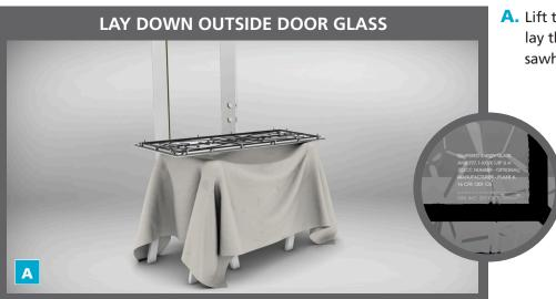
A. Lift the door off of the sawhorses and lay the outer frame with glass over the sawhorses.
