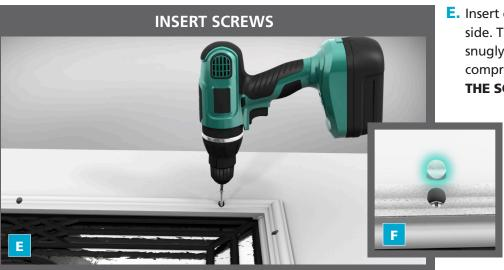
E. Insert each screw working from side to side. Tighten firmly so that the frame fits snugly against the door and the seal is compressed. AVOID OVER TIGHTENING THE SCREWS.
