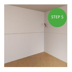
Install your plasterboard over the NuWave<sup>(m)</sup> Base and caulk the seams with an acoustic sealant to achieve the best results before finishing and painting your walls.
