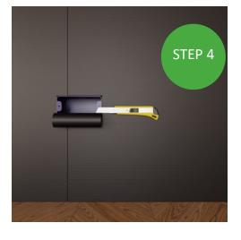
Use your cutting tool to carefully cut around outlet boxes as they become covered. Make these as close and as tight as possible to maintain a good seal.
