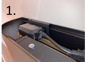
1. The remote receiver is attached to a black bracket with Velcro. This bracket is intended to attach to the back of the hood as shown. In this position the receiver will be just above the copper water distribution unit.
