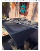
Step 8: Attached 5/8" Clear tubing to the ball valve and attach the ball valve to the ½" PVC, located inside the small oblique.
