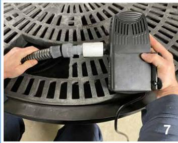
Set pump and hose in the basin. The fountain pump will be located beneath the pump access panel and inside the fountain basin. The pump should be positioned as close to the pump access opening as possible for best accessibility. This pump can be installed on its side, it will run in either position.
