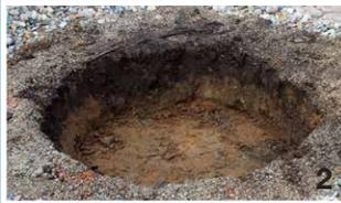
**NOTE:** If installing a splash apron, make sure the basin is about 1½" below grade, allowing you to slope the surrounding terrain toward the basin.
