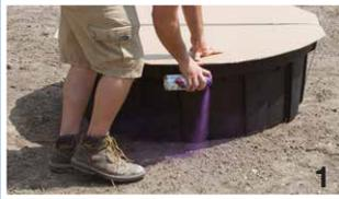
Clear the area and prepare to excavate by tracing the fountain basin using marking paint.
