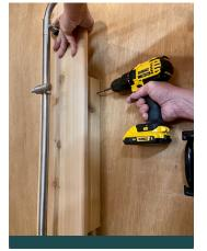
5. Screw shower mount to mounting board on both sides using 2" screws.
