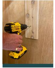
3. Screw mounting board to surface using 3" screws.
