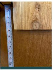
1. Place bottom edge of mounting board 42" from ground or floor.
