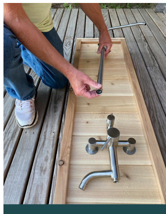
2. Check to be sure the rubber gasket is inside the end of the shower stem.
