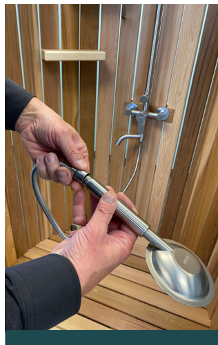
17. Attach the hand-held shower wand using sealing tape and gently tighten.
