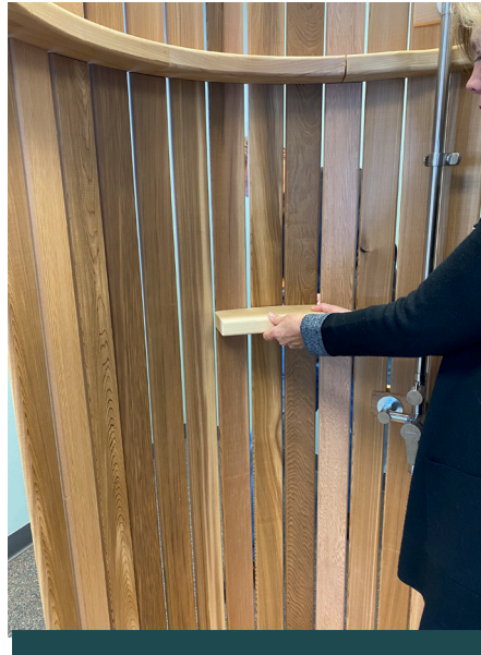
14. OPTIONAL: Install one or both of the shelves wherever desired. Use the level to ensure the shelf is straight and screw in place from the rear of the shower. NOTE: Have one person hold and level the shelf from the inside and another person attach from the back using two 2" screws.
