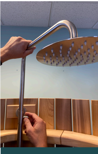
16. Adjust the height of the shower head using the lever as shown.
