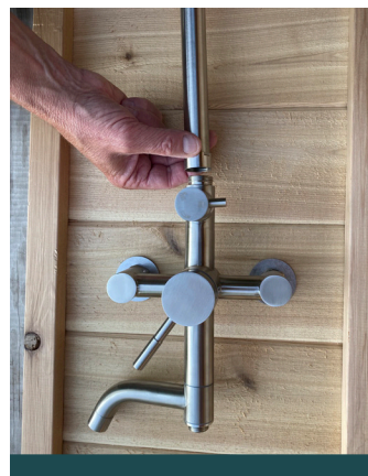
3. Hand tighten the shower stem onto the valve assembly (hand tighten only).
