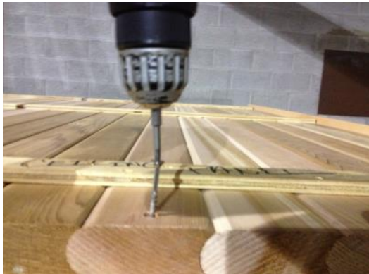
Fasten Roof Sections to Roof Support
