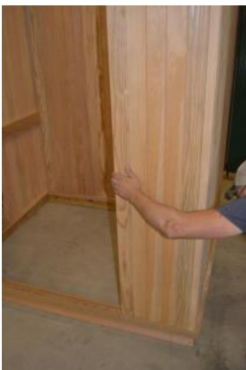
Position Wall Section F
