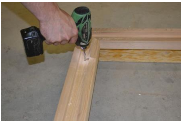
Fasten wall support rails to floor riser
