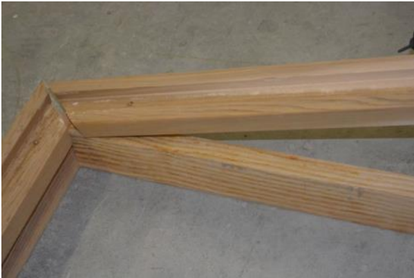
Position wall support rails
