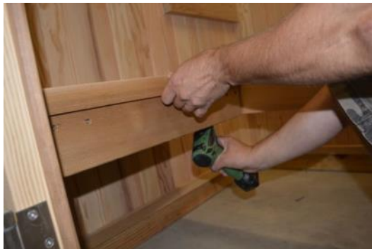
Attach Foot Rest and Lower Side Bench
