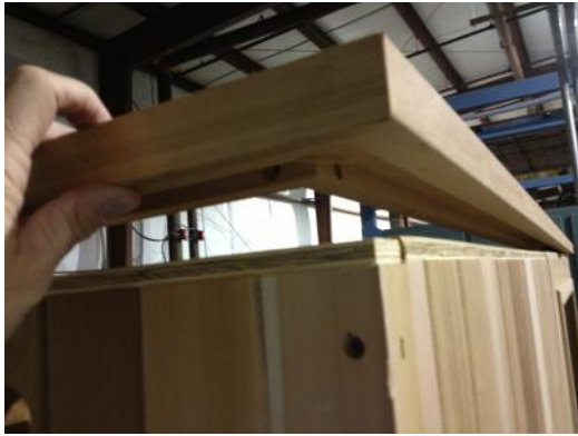
Attach Roof Support over walls
