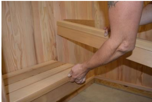
Attach Foot Rest and Lower Side Bench
