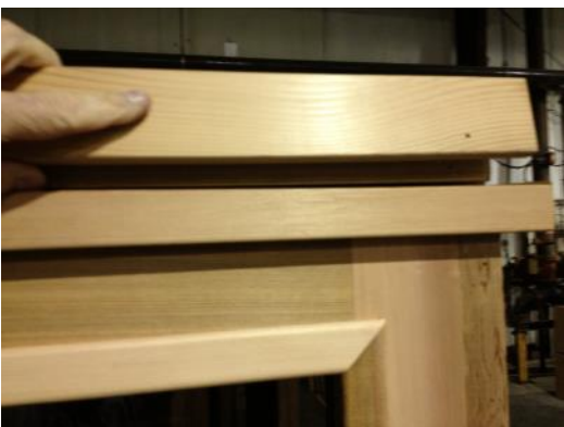
Attach Roof Trim pieces
