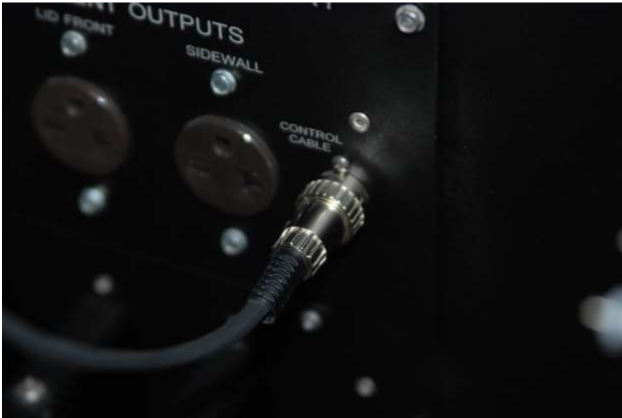
Figure 53- Re-install Control Cable
