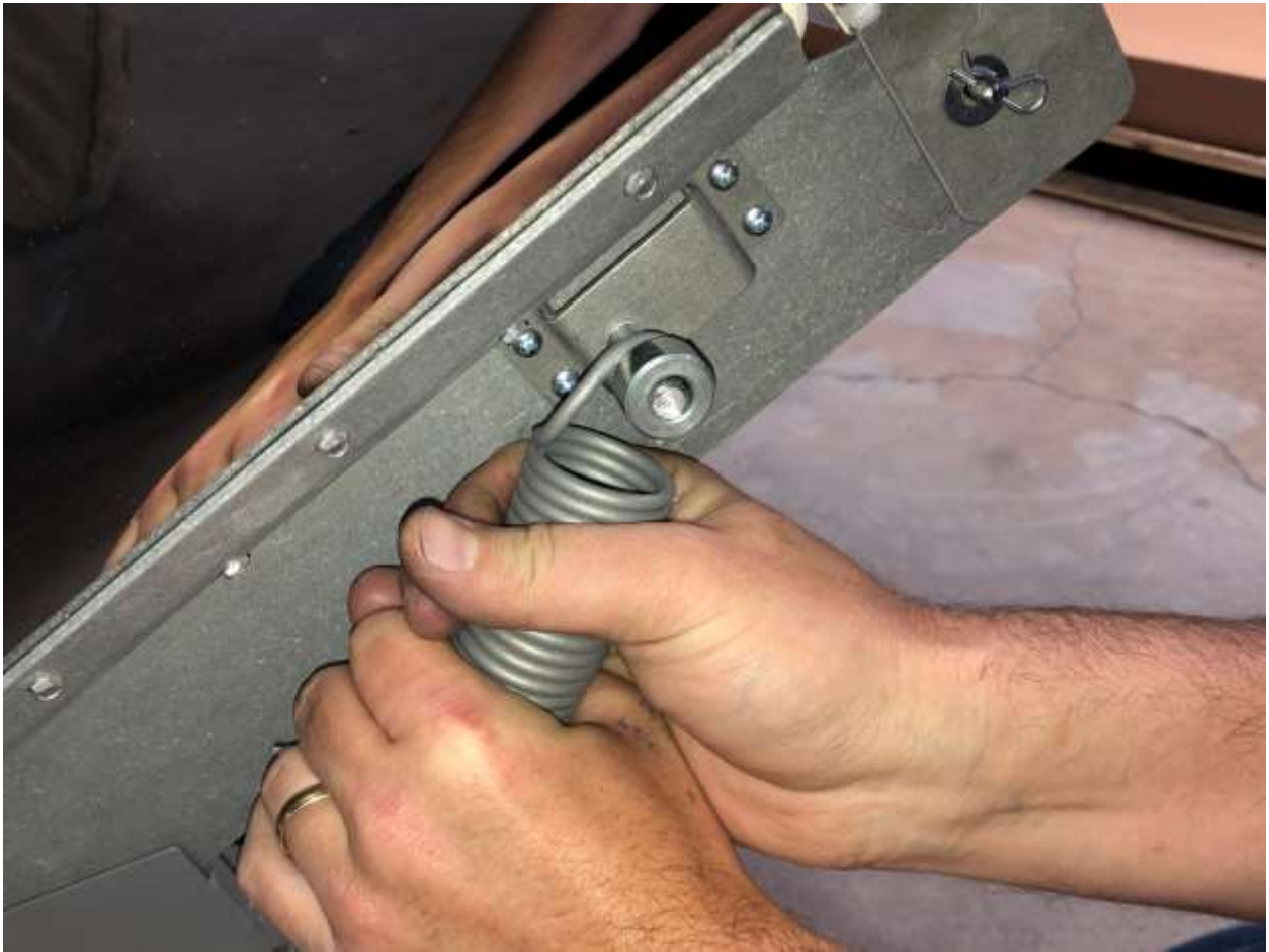
Figure 83 - Lift Assist Spring Installation SP28 and SP41
