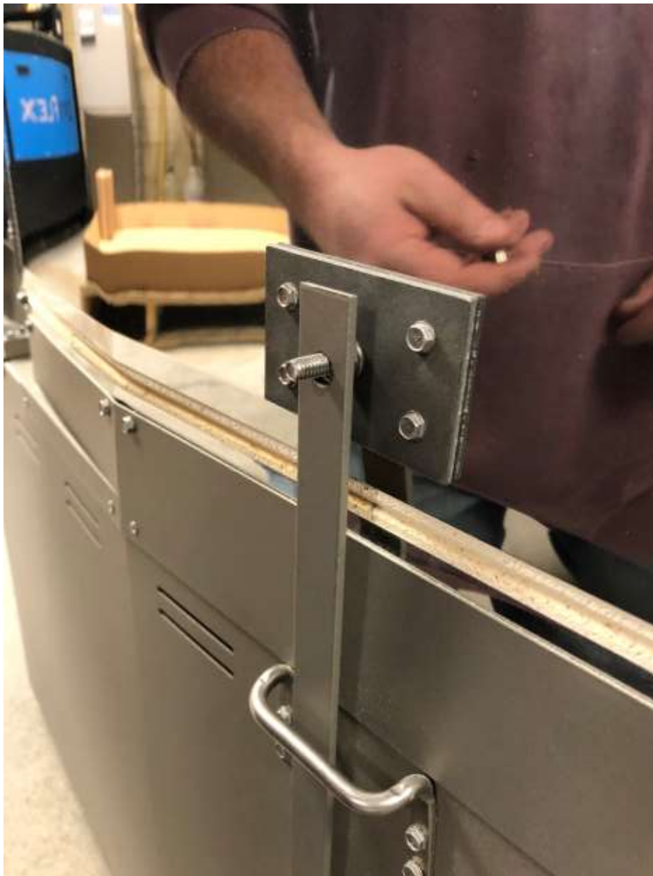
Figure 75 - Chamber Safety Bar Installation
