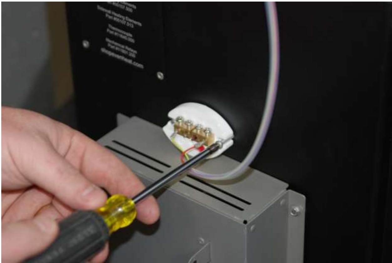
Figure 52 - Fasten the Thermocouple
