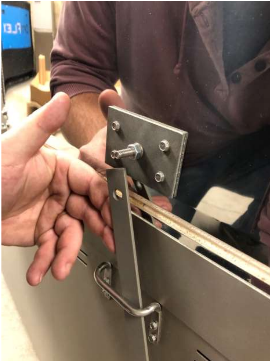
Figure 74 - Chamber Safety Bar Installation
