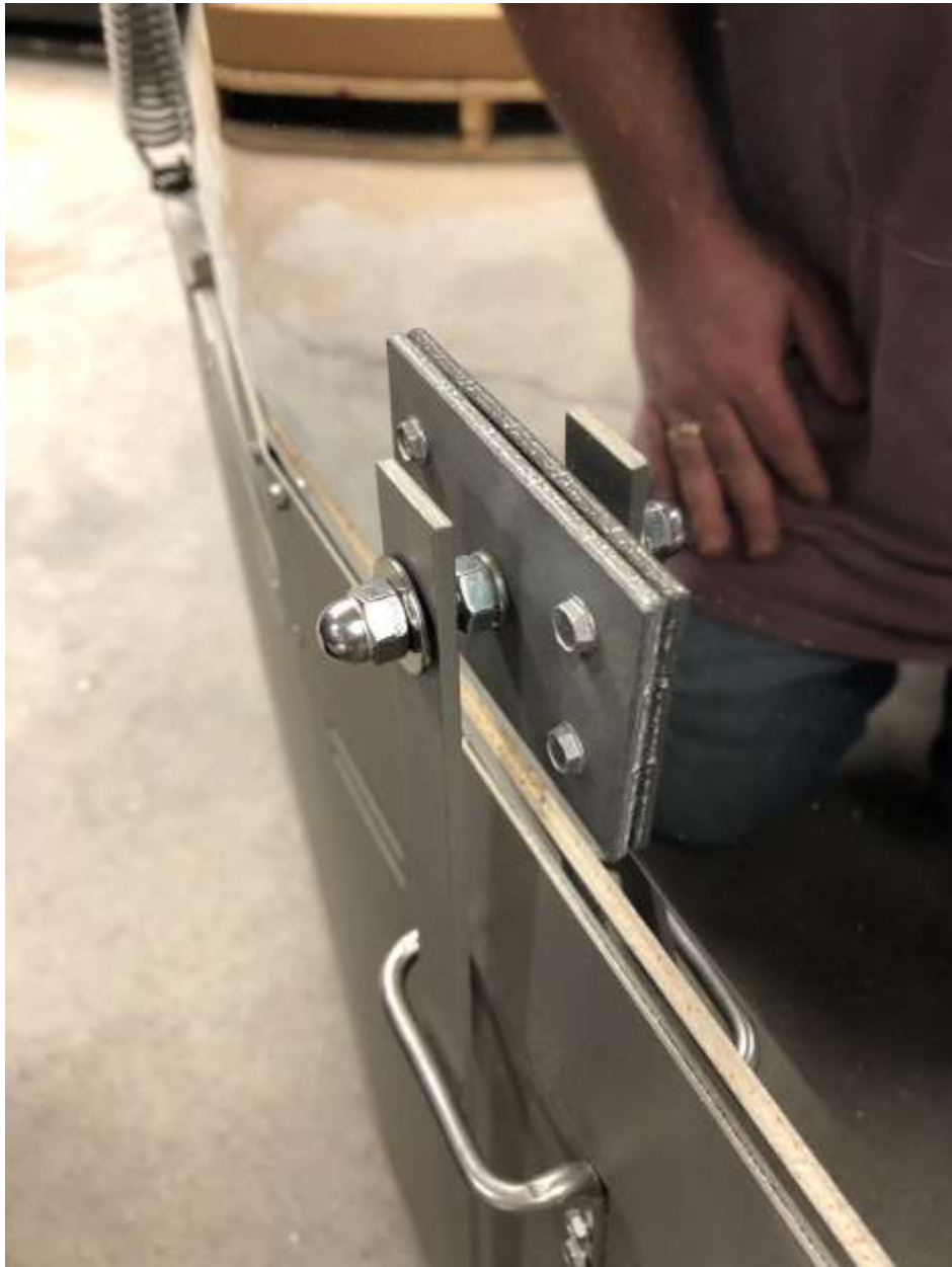
Figure 77 - Chamber Safety Bar Installation
