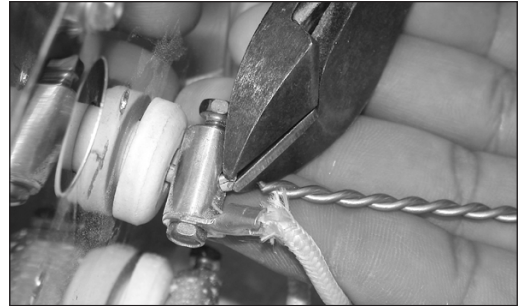
Tighten the element connectors according to step #14. Then cut off the element ends.
