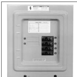
Know the location of the circuit breaker panel. Label the breaker that controls your kiln's circuit.
