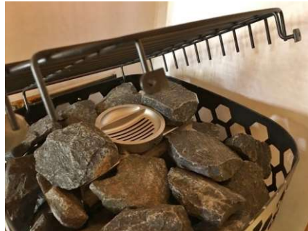
BWT tank, tank lid, and the vent cover installed and the rocks placed around the tank.
