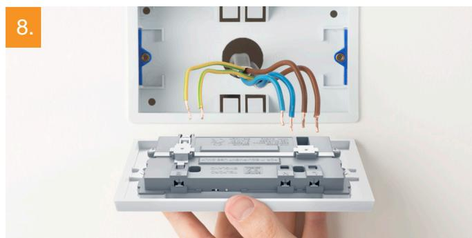
8. Line up the new socket and take note of where each terminal is located.
