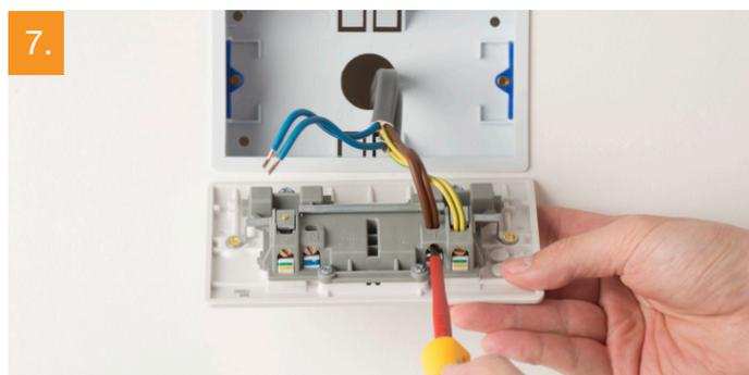
7. Whichever wiring configuration you find, unscrew each terminal screw to release the wires. You should now be able to remove the socket and place it to one side.
