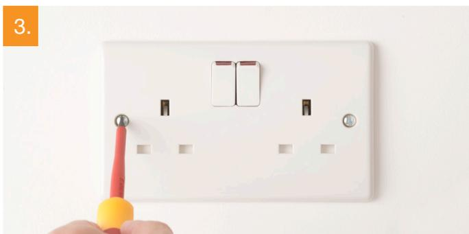
Test power is not supplied to the socket by using a plug in socket tester or multimeter. Unscrew the retaining screws on the socket so that it is released from the mounting box.
