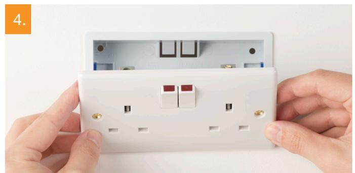
Gently ease the socket from the mounting box to show the wiring.
