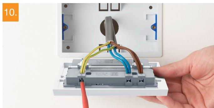
10. Make sure that the wires are fully inserted into the terminal and that no bare copper wire is visible. Tighten the screws securely onto the copper wire, not the outer sheathing.
