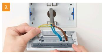
Place the blue wire(s) into the neutral terminal, brown into the live terminal and green/yellow into the earth terminal. The terminals on the socket are colour-coded to help locate the correct one.
