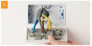
There will generally be three different wiring configurations. This photo shows a single wire of each colour connected to each terminal.
