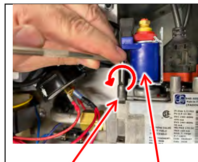
MANIFOLD PRESSURE TAP
