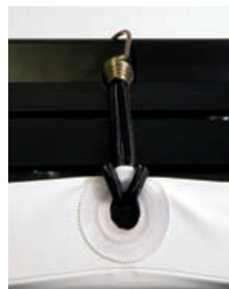
▲ Elastic stretchers and eyelet detail
