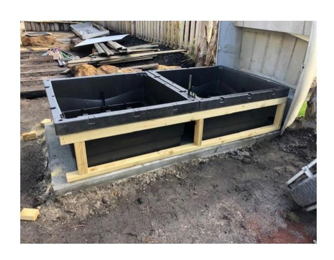
Clad with blue board or cement sheet, 450mm eave sheets are good. If you set the frames up just back from the top lip when you screw the blue board on it finishes flush with the top lip on the Foodcubes
