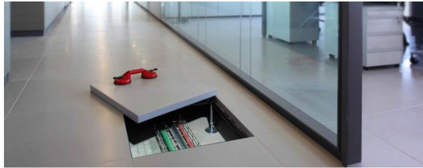
RAISED ACCESS FLOORING FOR PLUMBING & ELECTRICAL
