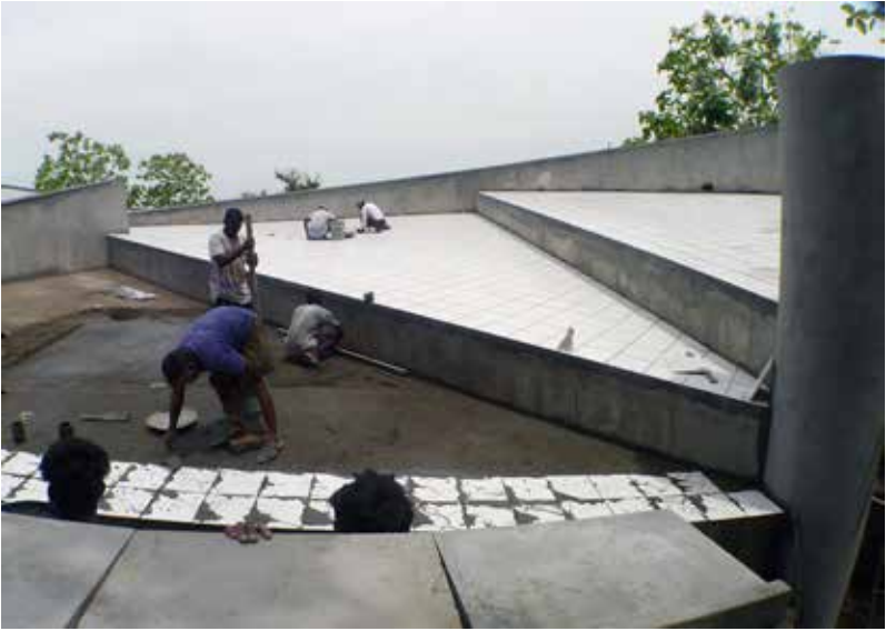
Tiling the roof of the Sangam Hall, September 2016
