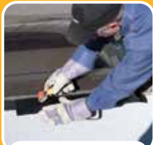
Built Up Roof
