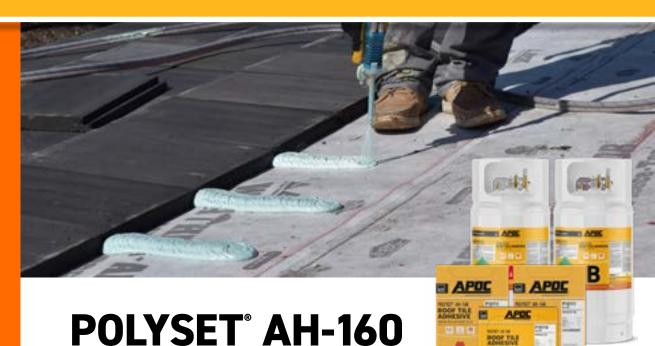
APOC Polyset AH-160 is a two-component, low pressure spray polyurethane foam adhesive that adheres each individual tile in place with superior holding power compared to nails, screws, mortar
