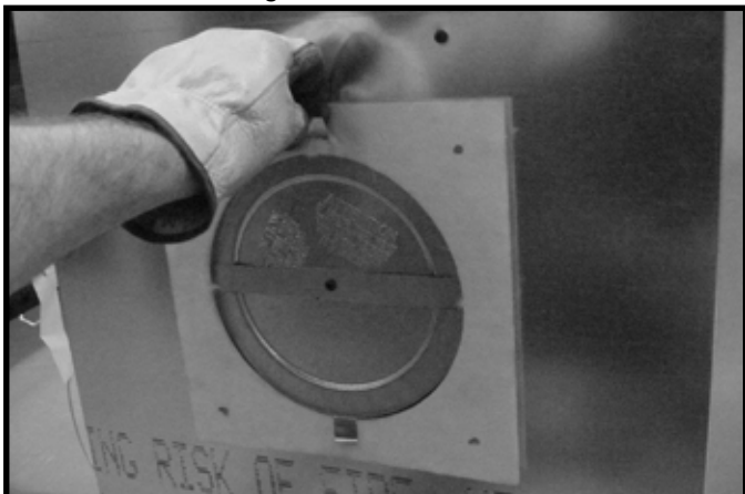
Figure 6.8 (Generic Fireplace Shown) Fold the tabs toward the center of the fire plug (90°) and remove the insulation gasket.
