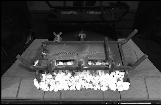
Figure 11.11. Teco-Sil Placement
