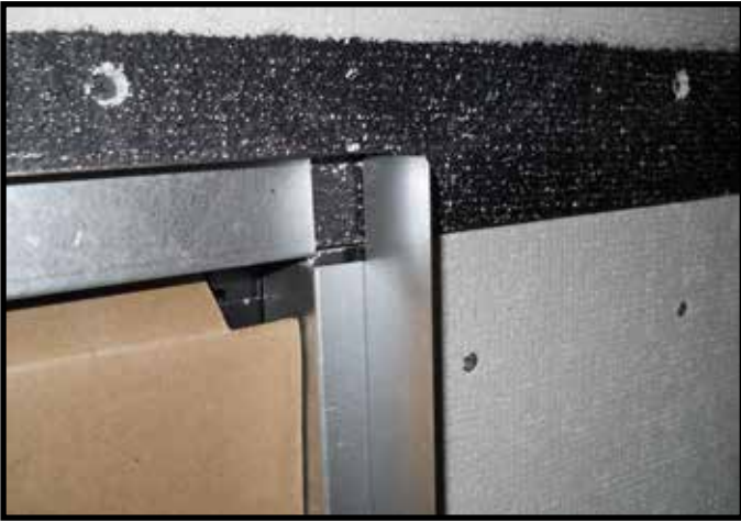
Figure 10.5 Finishing Template Bends
