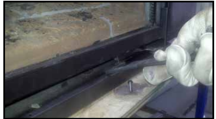
Figure 11.2. Glass Clip Tool Location
