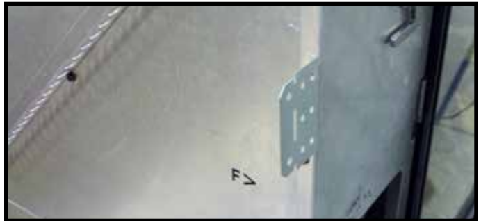
Figure 6.4 Nailing Tab Bent Out for Installation
