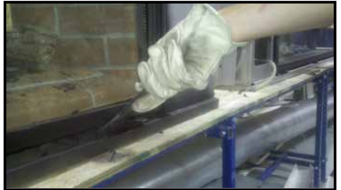
Figure 11.3. Inserting Glass Clip Tool
