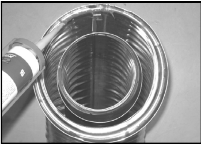
Figure 7.1 High Temperature Silicone Sealant
