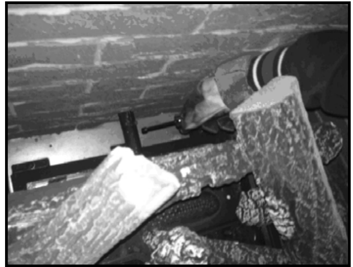
Figure 9.1. Air Shutter Location
