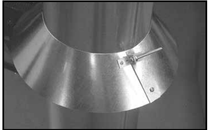
Figure 7.12 Insert Bolt into Brackets
