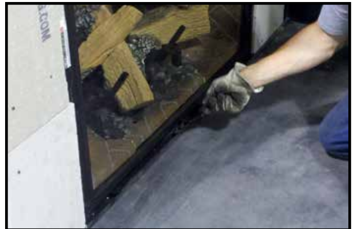
Figure 11.8. Securing Bottom Glass Clips
