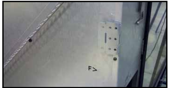
Figure 6.3 Side Nailing Tab in Shipping Position
