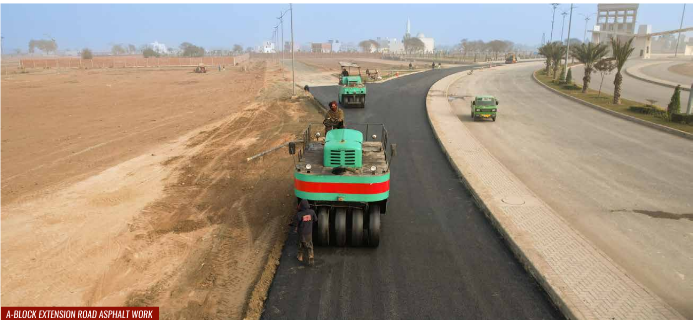
A-BLOCK EXTENSION ROAD ASPHALT WORK
