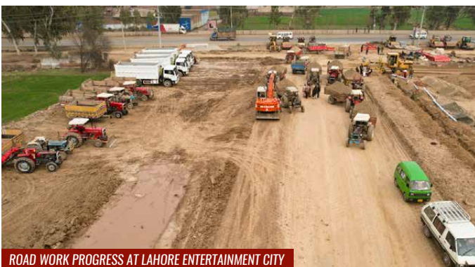
ROAD WORK PROGRESS AT LAHORE ENTERTAINMENT CITY
