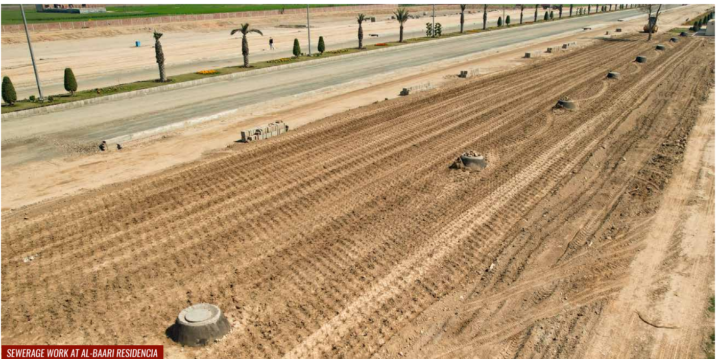
SEWERAGE WORK AT AL-BAARI RESIDENCIA
