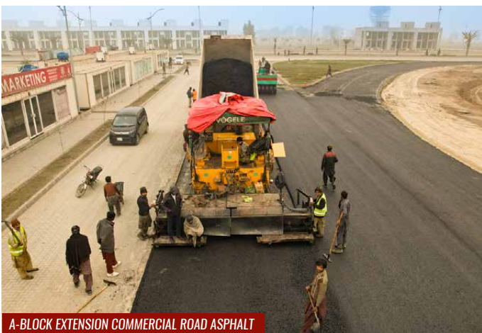
A-BLOCK EXTENSION COMMERCIAL ROAD ASPHALT
