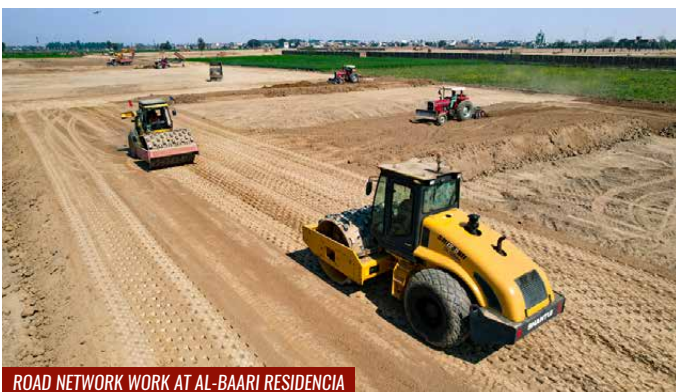
ROAD NETWORK WORK AT AL-BAARI RESIDENCIA
