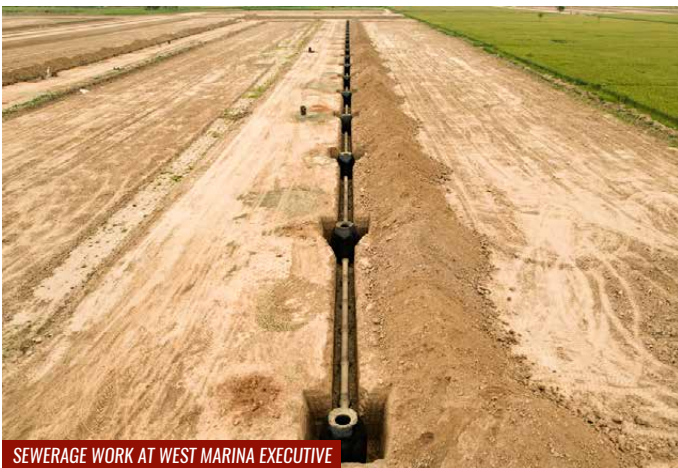
SEWERAGE WORK AT WEST MARINA EXECUTIVE
