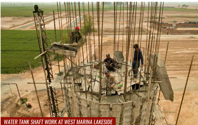
WATER TANK SHAFT WORK AT WEST MARINA LAKESIDE
