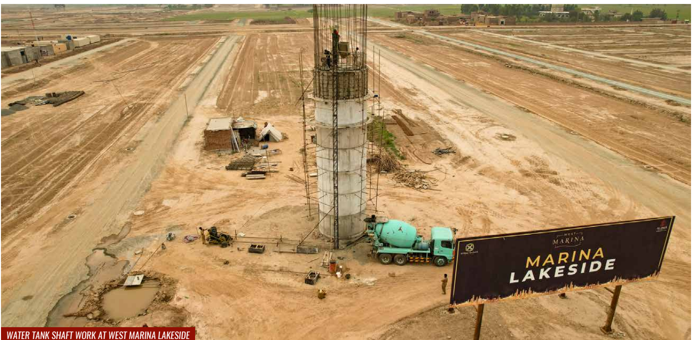
WATER TANK SHAFT WORK AT WEST MARINA LAKESIDE
