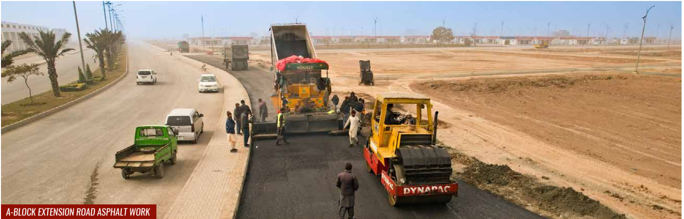
A-BLOCK EXTENSION ROAD ASPHALT WORK
