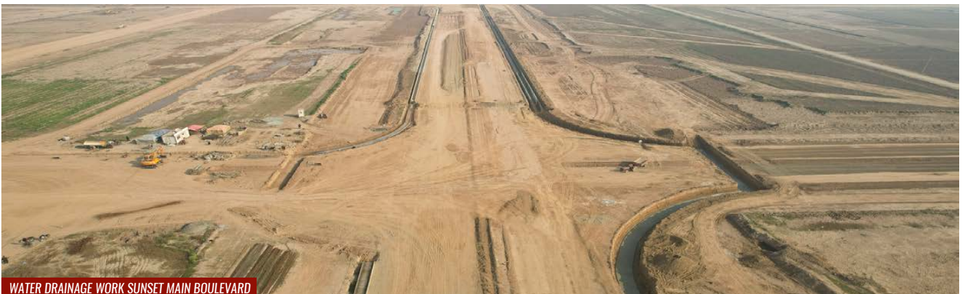
WATER DRAINAGE WORK SUNSET MAIN BOULEVARD
