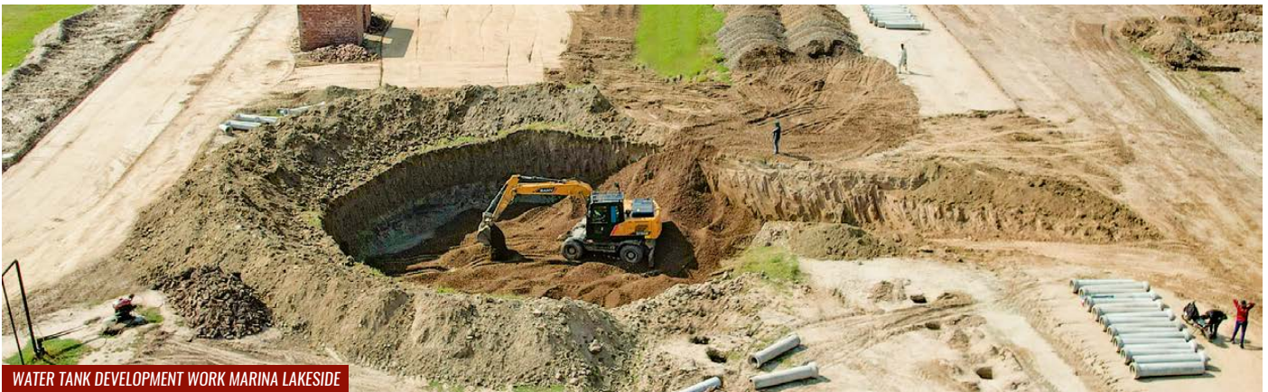
WATER TANK DEVELOPMENT WORK MARINA LAKESIDE
