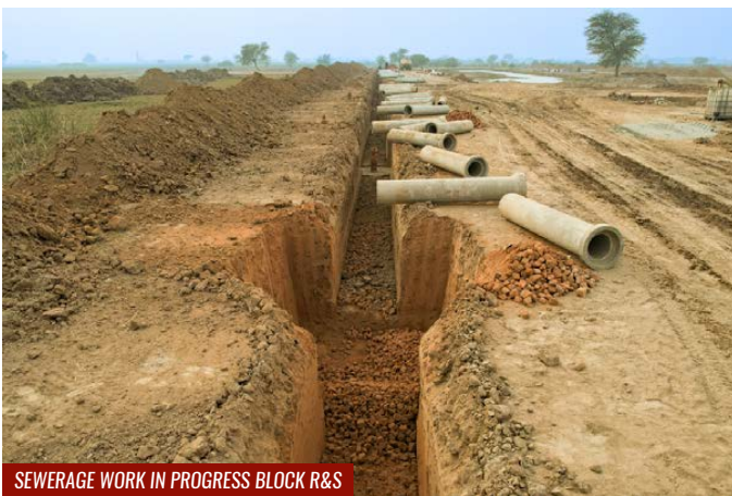
SEWERAGE WORK IN PROGRESS BLOCK R&S
