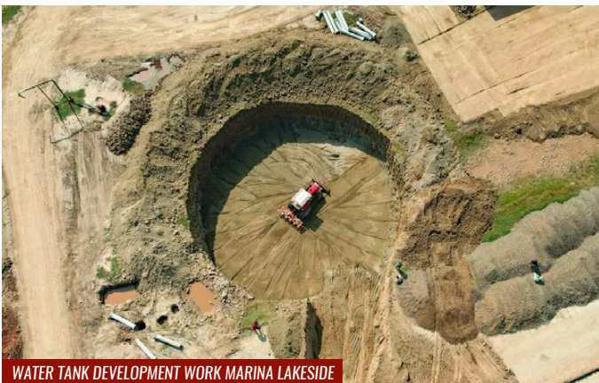
WATER TANK DEVELOPMENT WORK MARINA LAKESIDE
