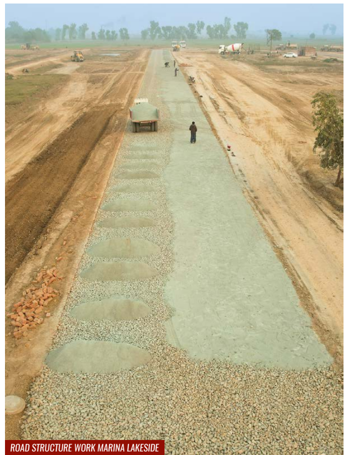
ROAD STRUCTURE WORK MARINA LAKESIDE
