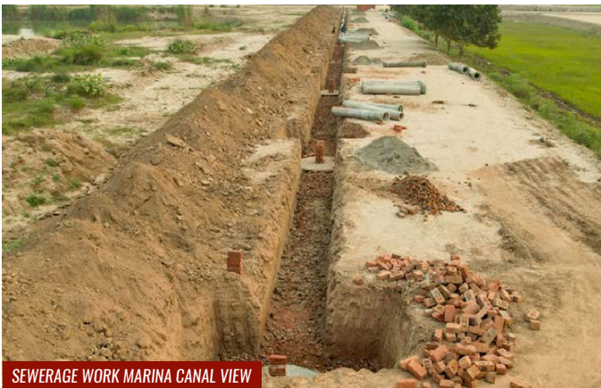
SEWERAGE WORK MARINA CANAL VIEW
