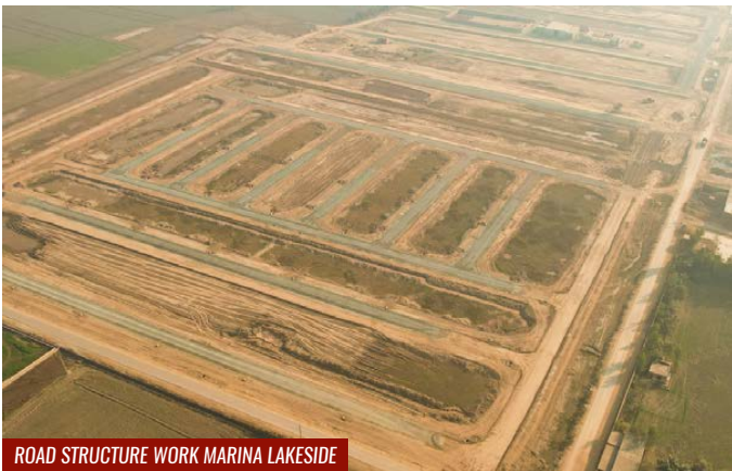
ROAD STRUCTURE WORK MARINA LAKESIDE
