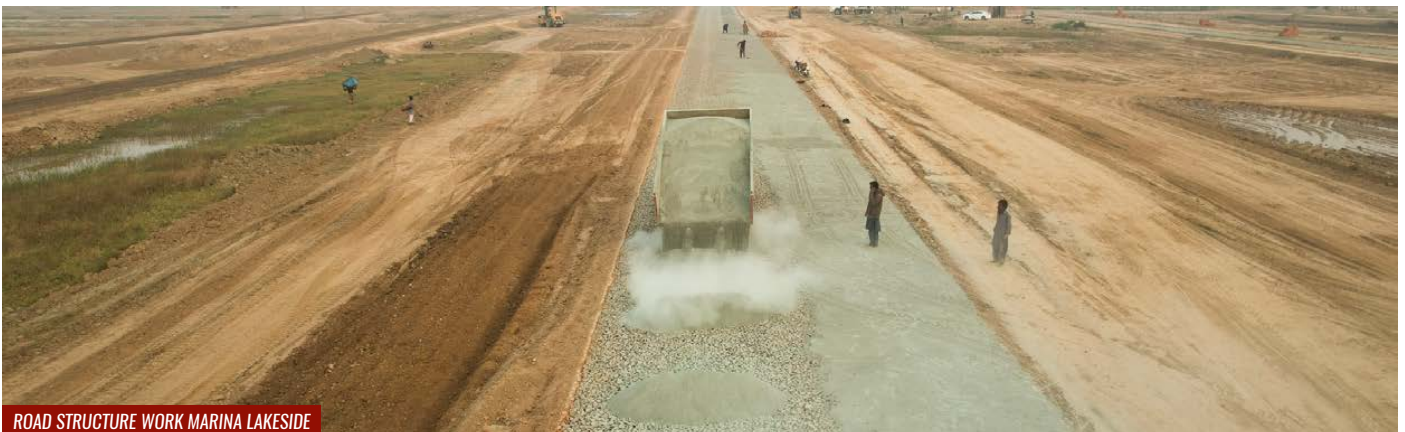
ROAD STRUCTURE WORK MARINA LAKESIDE
