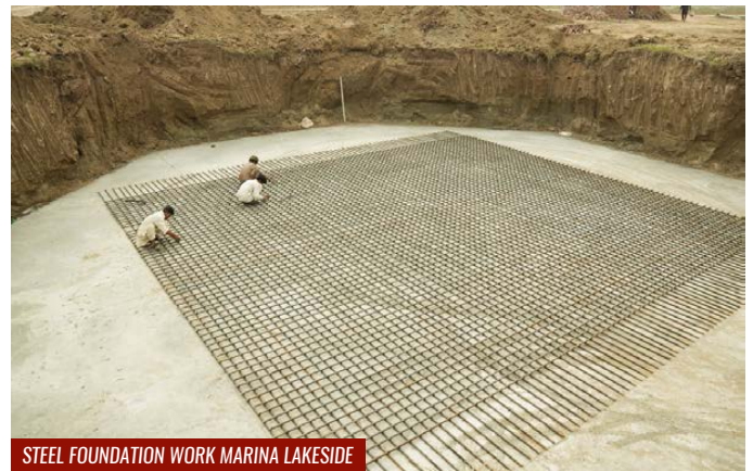
STEEL FOUNDATION WORK MARINA LAKESIDE
