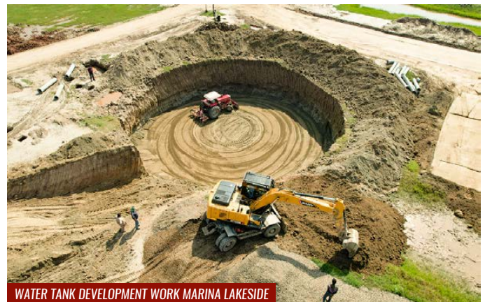
WATER TANK DEVELOPMENT WORK MARINA LAKESIDE
