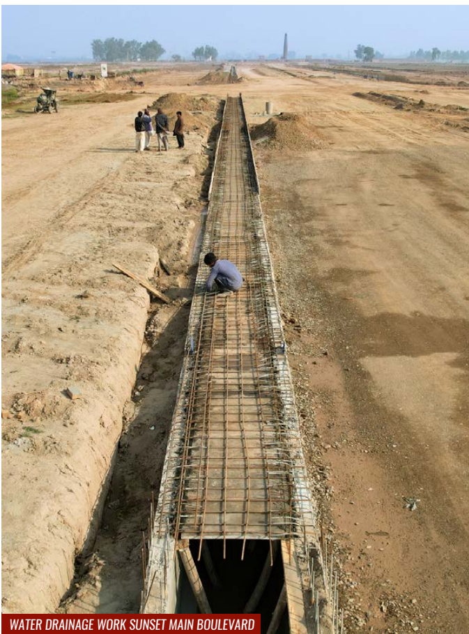
WATER DRAINAGE WORK SUNSET MAIN BOULEVARD
