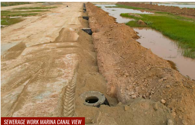
SEWERAGE WORK MARINA CANAL VIEW
